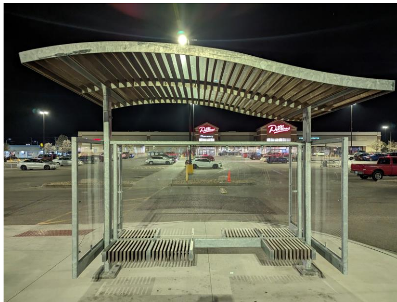
Figure 21 - Bus stop bench
