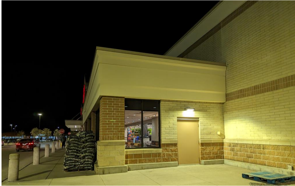
Figure 18 - Dillons utility door
