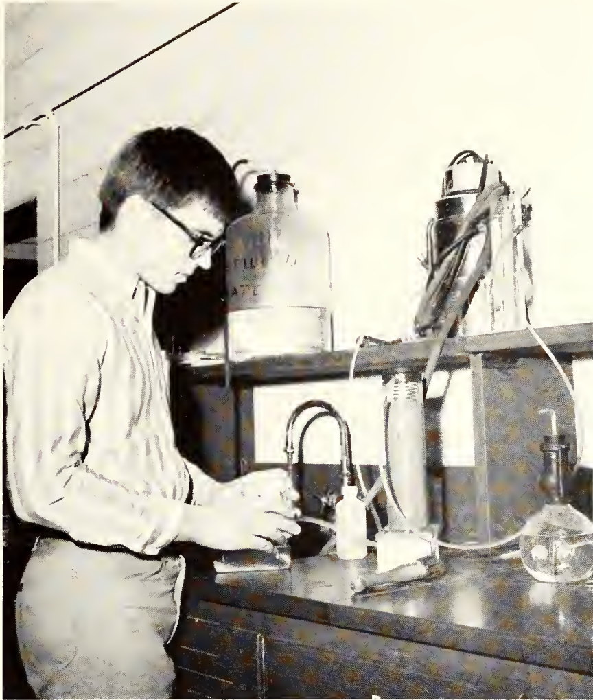
Soil samples are classified for use in construction jobs for highways and railroad beds by students in Soil Mechanics I.
