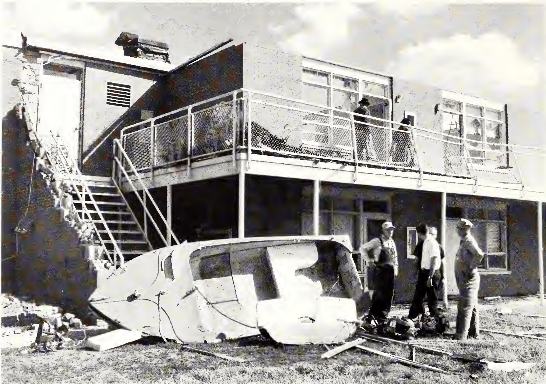
Forced to evacuate after a June 8 tornado caused extensive damage to Jardine apartments, married students move to tem-
