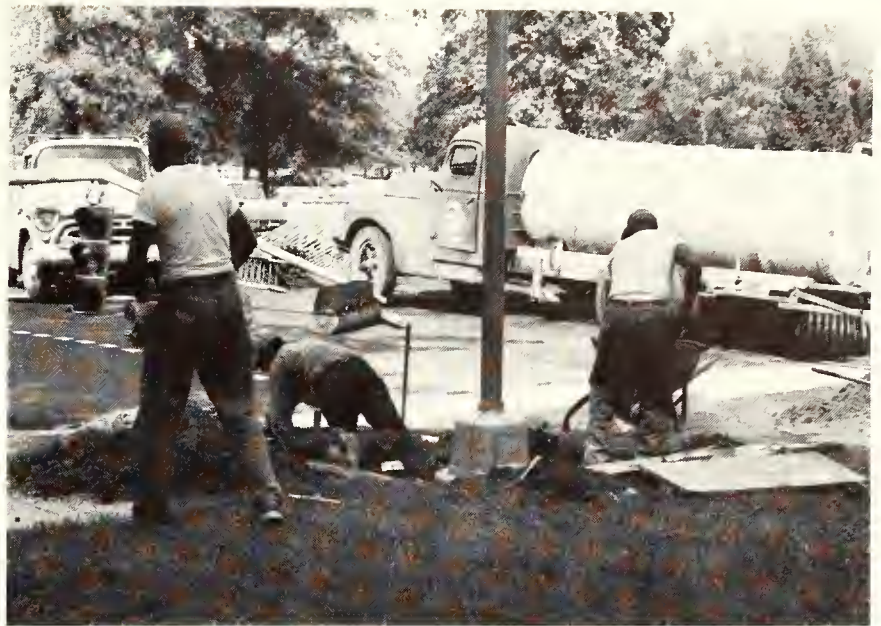
Workmen labor during August to complete a street cutoff by-passing Aggieville to help relieve campus traffic congestion.
