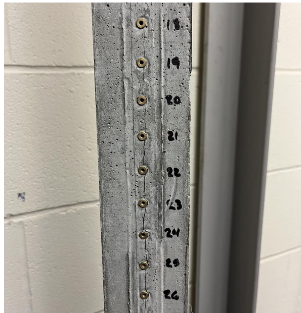
Figure 26. Cracked test specimen used for UHPC 27% test
