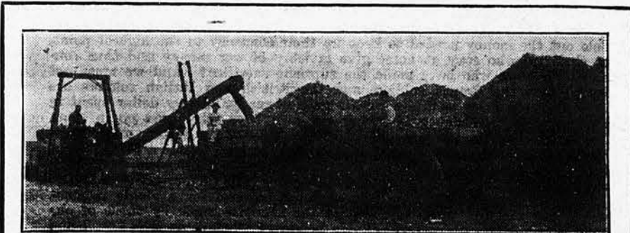
UNLOADING CORN IN DICKINSON COUNTY WITH MOVABLE ELEVATOR— A GREAT LABOR-SAVER
