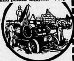
Besides doing all ordinary work, Cushman Engines may be easily attached to machines in field. Picture shows 8 H. P. on Hay Baler.
