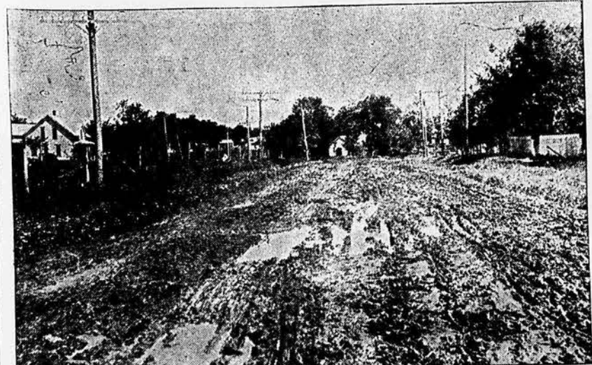
SCENE ON RED LINE ROAD.—RESULTS OF POOR DRAINAGE
