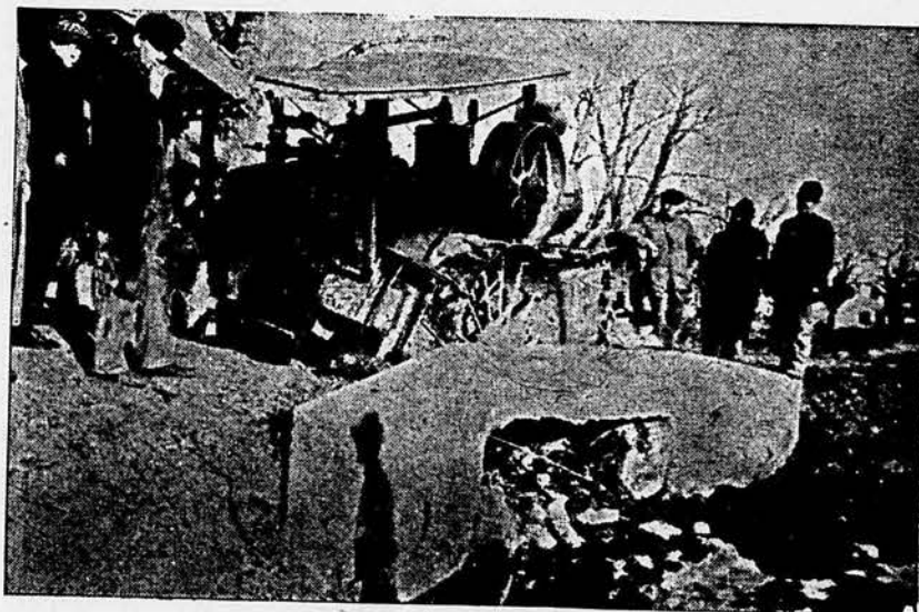
THIS IS WHAT HAPPENS TO IMPROPERLY DESIGNED CULVERTS
