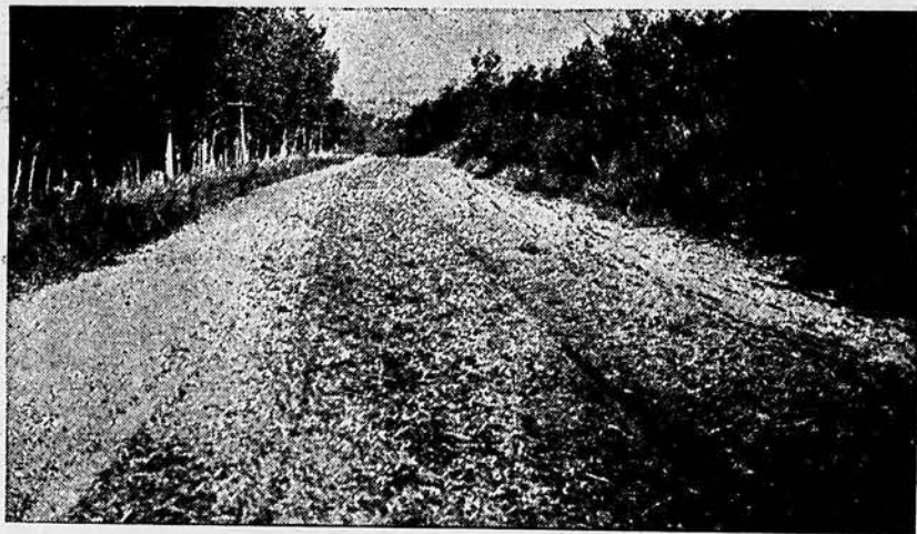
SAND ROAD IN RILEY COUNTY COVERED WITH STRAW
