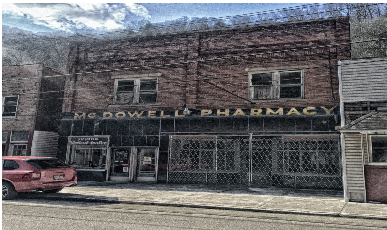
Figure 4.11. A photo taken outside of the former McDowell Pharmacy building. The business has been shut down and the building boarded up due to increasing health and safety concerns.
