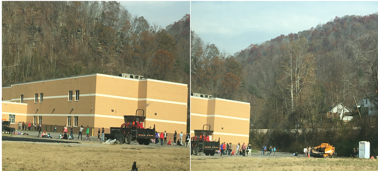
Figure 4.9. Photos taken outside of the Southside K-8 Community School during recess. Unused construction equipment and a portable toilet remain at the site of what was once the construction area of the school's playground.
