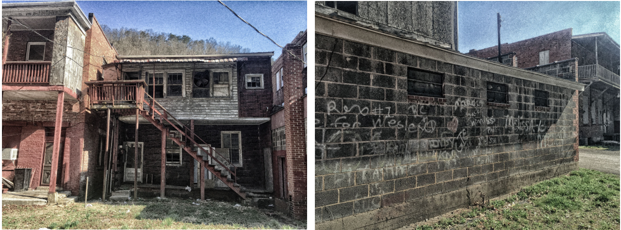
Figure 4.13. Graffiti lines the outside of an abandoned building in McDowell County—some of which notes messages of violence from one community and/or familial group to another.
