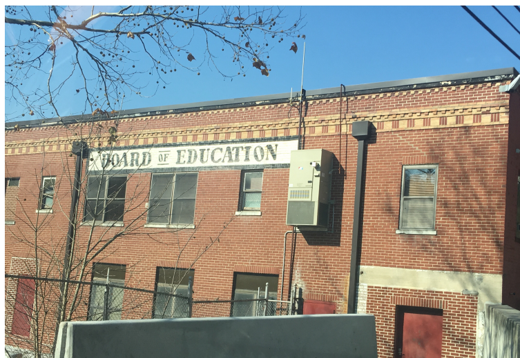
Figure 4.8. A photo of the outside of The McDowell County Board of Education building, located in the county seat of Welch, West Virginia.
