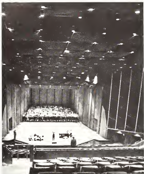
Auditorium acoustics can be changed by moving the walls and ceiling.
