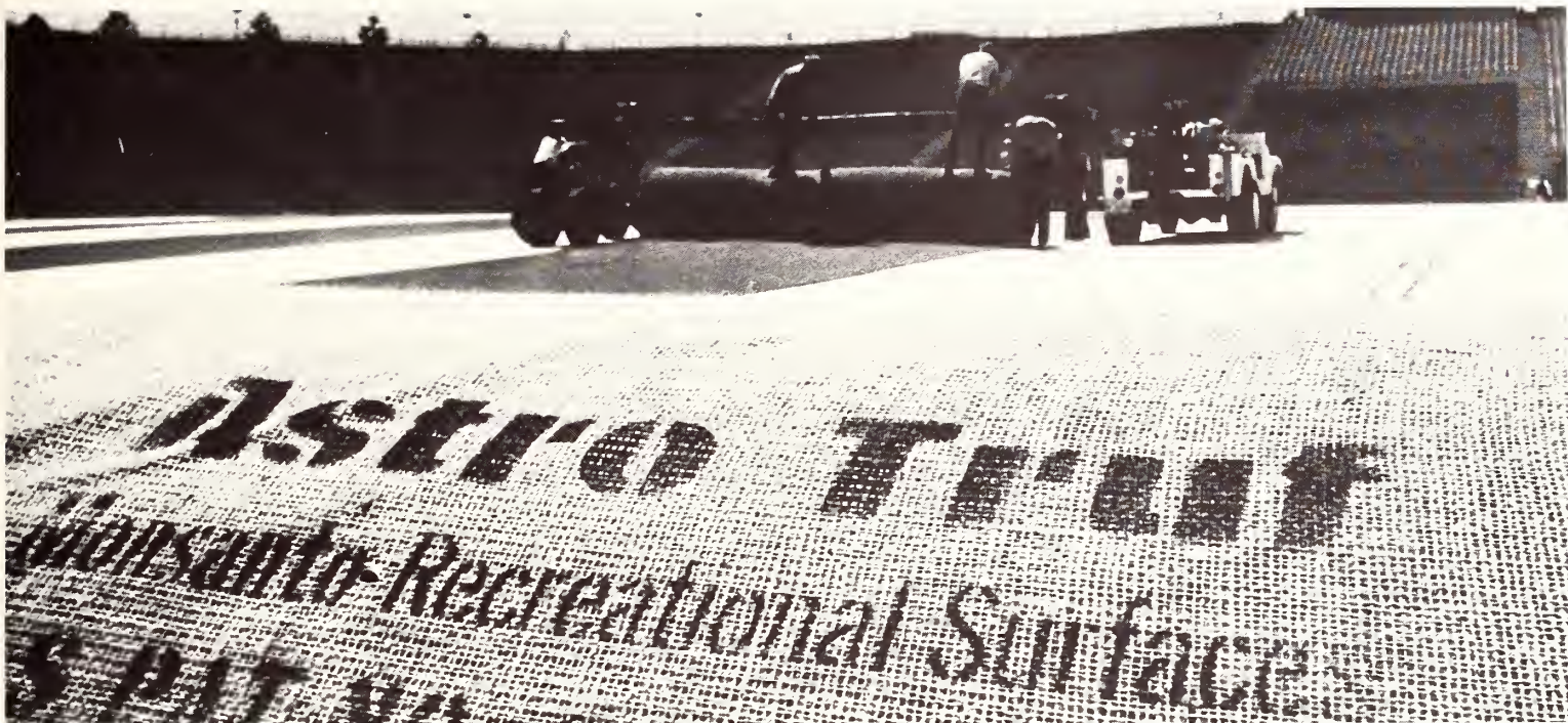
Monsanto workmen install artificial turf on the playing field of
