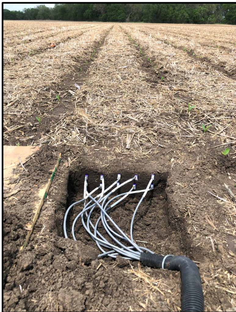
Appendix Figure A-1 HP probe installation in the inter-rows of corn.
