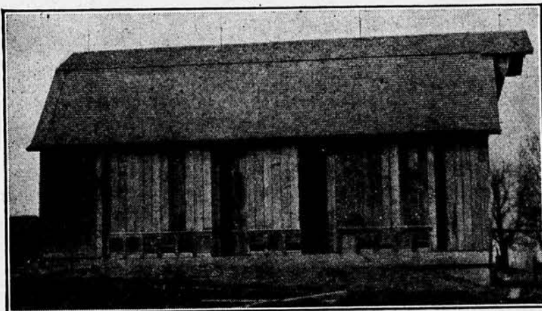
H. M. Lefever, Chanute, Has One of the Finest Jersey Herds in the State, and Milks 20 to 25 All Year. This Barn Is One He Built During Pleasant Days Last Winter, Out of Used Lumber. A 5½-Foot Concrete Foundation Forms Part of the Wall of Basement Where Cows Are Housed. Chutes Carry the Feed and a Single Handle Opens and Closes Stanchions
