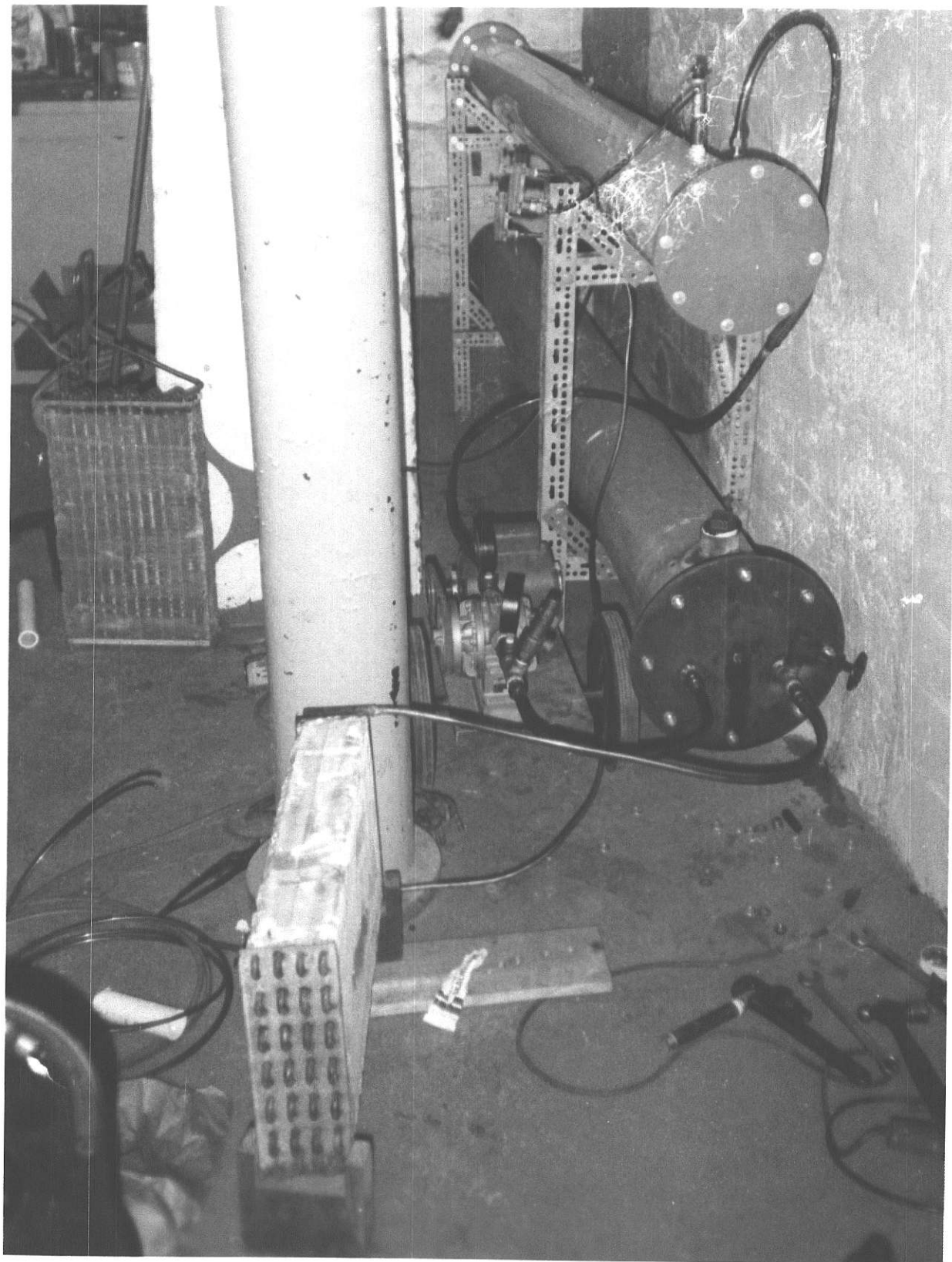
Figure 14: Distillation tube, (top), boiler, (middle), and auxiliary heat exchanger, (bottom), early in construction.
