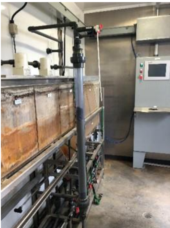
Figure B.5 Ion-Exchange Column
