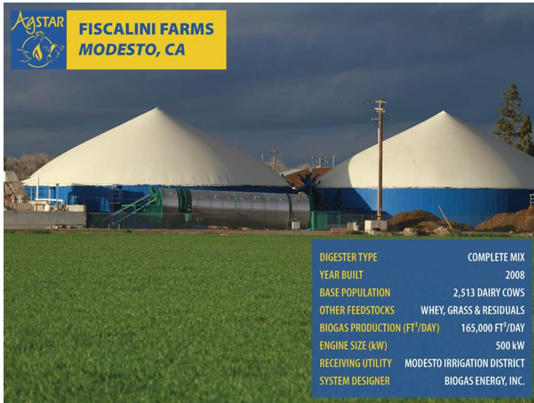
Figure A.2 Above Ground Complete Mix Digester
