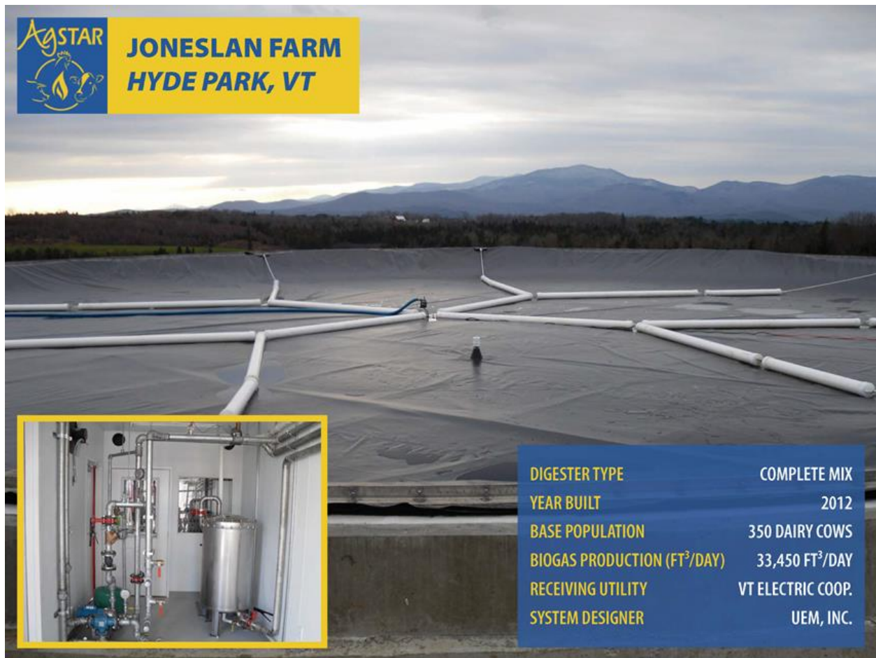
Figure A.3 Below Ground Complete Mix Digester
