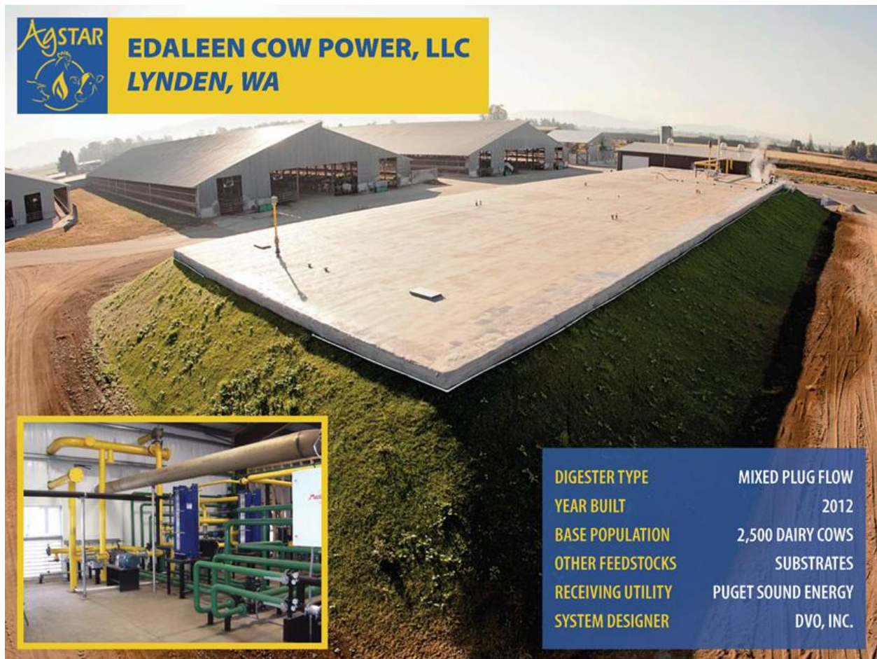
Figure A.4 Below Ground Mixed Plug Flow Digester
