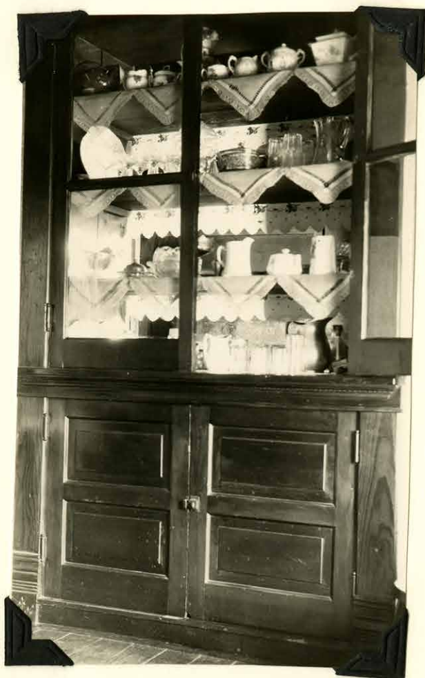
Fig. 30-Anpass cupboard from Mrs. Huff's dining room to the pantry. This cupboard illustrates a waste of space. The shelves could be made adjustable and the space between them reduced. Additional shelves could thus be added to make room for more storage.
