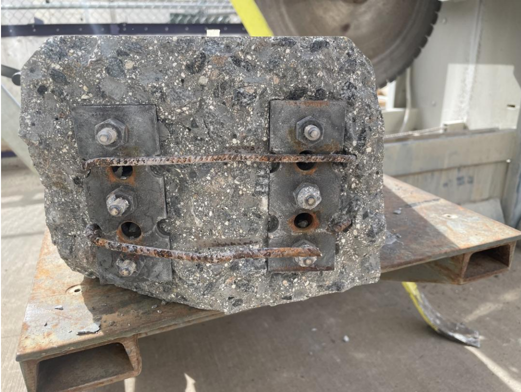
Appendix A Figure 16: Results from Dry Cutting PT Tie at End
