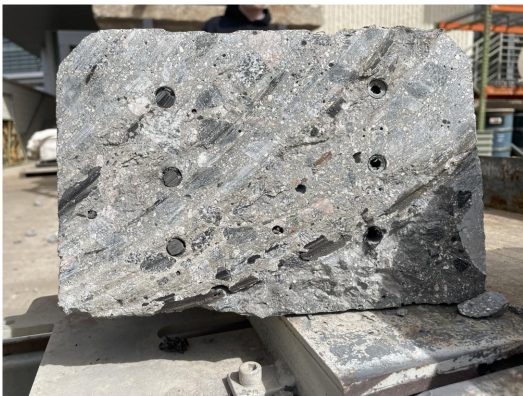
Appendix A Figure 15: Results from Dry Cutting PT Tie at Cut
