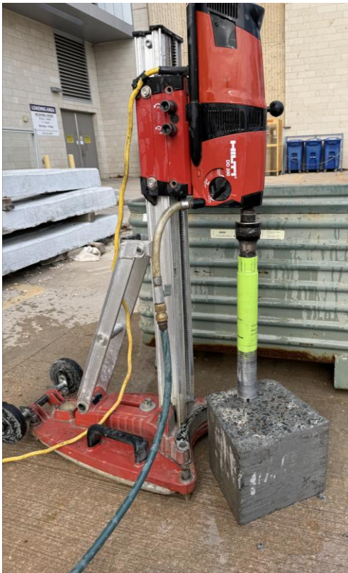
Figure 9: Concrete Coring Rig
