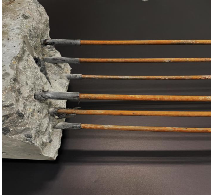
Figure 31: Corrosion at Midspan
