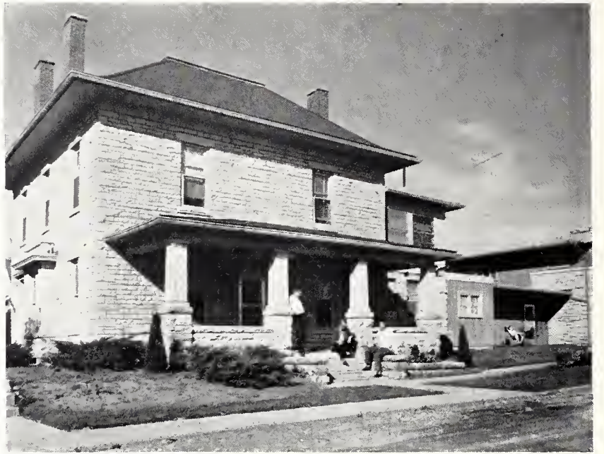
REPAINTING the interior and adding a new roof were major changes made at the ATO house, 1408 Denison.
