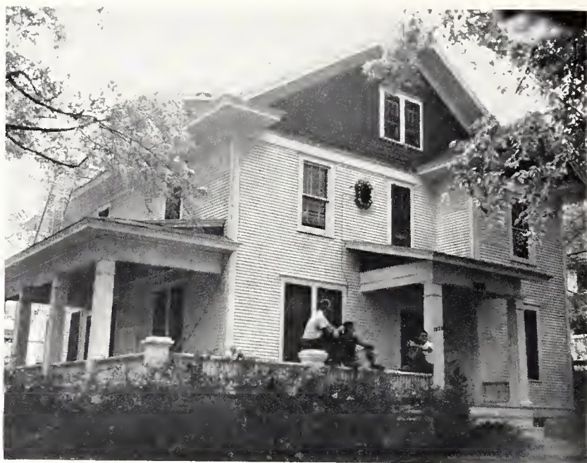
WITH THE removal of part of the porch, the Phi Kappa Tau house, 1623 Fairchild, has a bigger front lawn.
