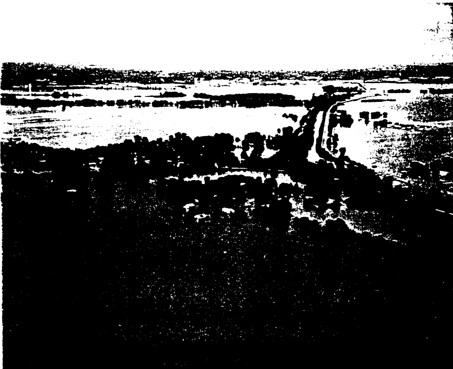
Figure 2.1: Aerial view of Mississippi River flooding along Highway 367, West Alton, Illinois (Cover photo, K.L. Wahl, K.C. Vining, G.J. Wiche, 1993).
