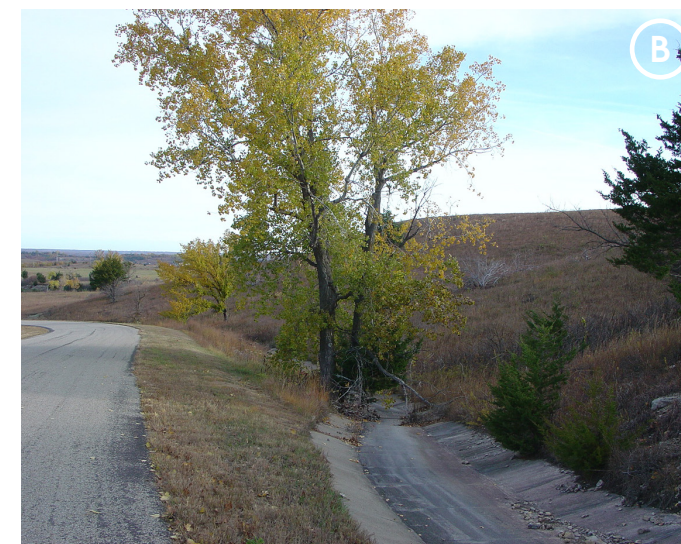
Figure 3.38 View of Road Along Top of the World Drive (Skabelund 2006)
