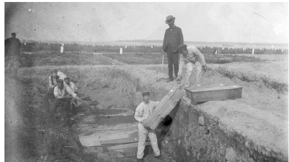
Figure 2.21 A trench at the potter's field on Hart Island, NY (Riss, circa 1890)
