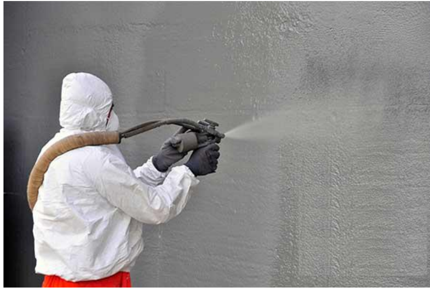
Figure 11. Carbonation Barrier Coatings Application (Constro Facilitator, 2021)
