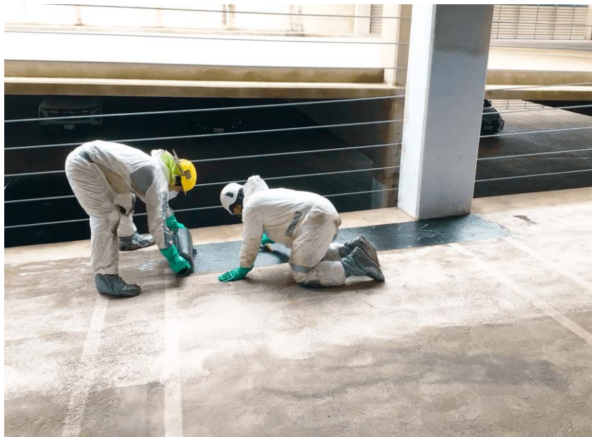
Figure 17. CFRP Strengthening of Concrete Slab (DYWIDAG, N,d,)
