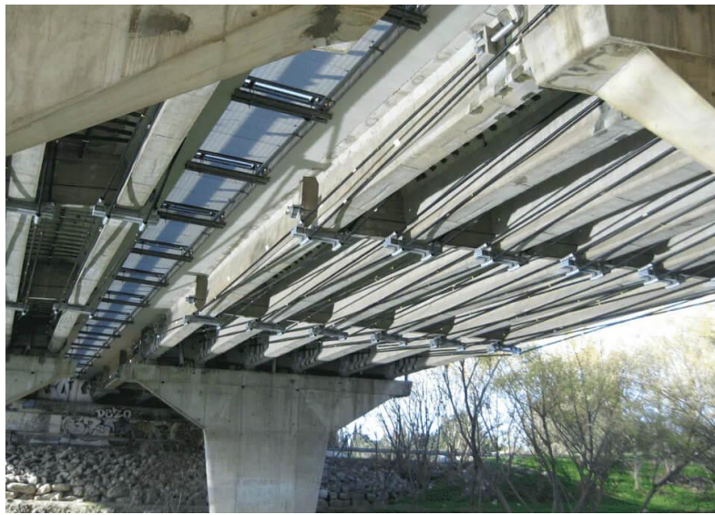
Figure 15. External Post-Tensioning of Concrete Bridge Beams (Freyssinet, N.d.)
