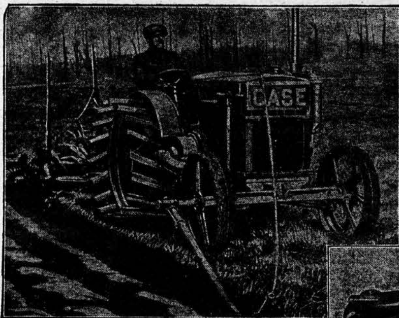
Illustration shows Case 10-18 Kerosene Tractor pulling 2-bottom Grand Detour Plow.
