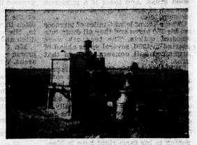
Above: This deep-well turbine pump is located on the T. L. Welsh farm, east of Abilene. Pressure direct from the well is used to force water thru the sprinkler system for alfalfa production in dry years.
