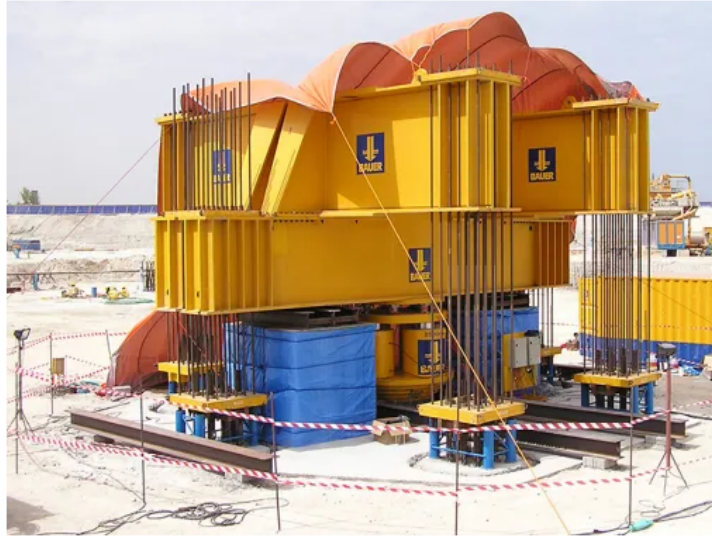
Figure 29: 6000 Ton Pile load test setup (The Constructor, n.d.)
