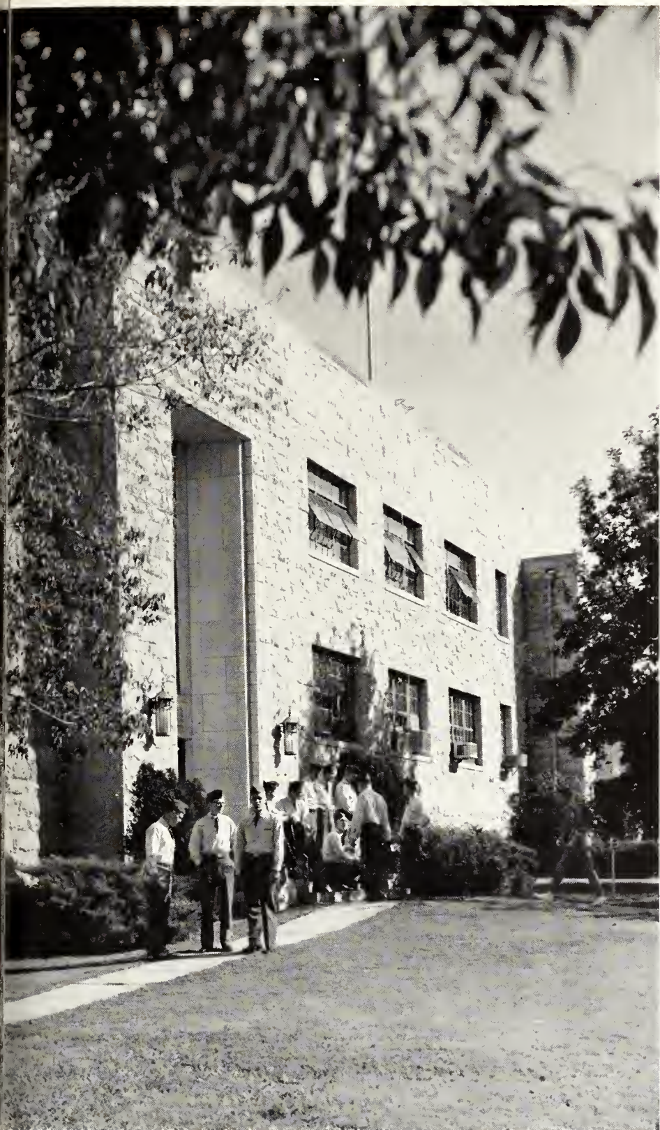
ARMY AND AIR Force ROTC detachments, more than 1,500 strong, are located in the Military Science building.
