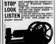
(Patented May 15, 1906.) The only horizontal, vapor cooled gasoline engine in the world. Worth twice the price of any other style gasoline engine, but costs you no more. Illustrated
