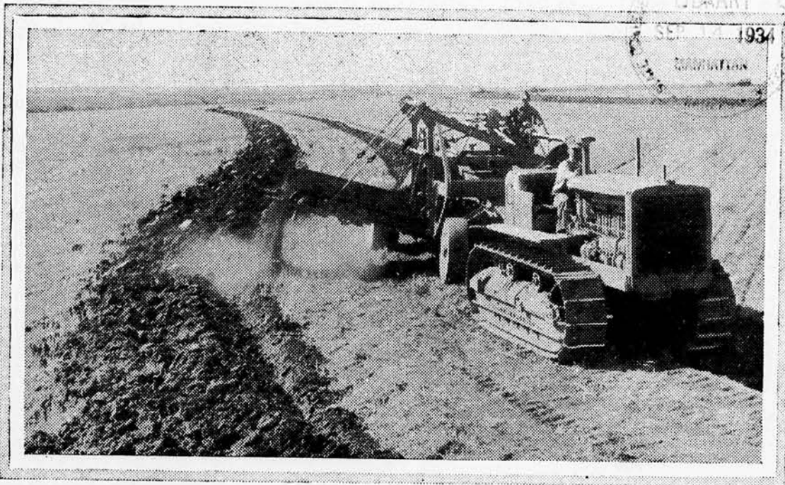
Caterpillar Diesel 50 and Caterpillar power-controlled elevating grader equipped with short carrier, building terraces on the U. S. soil erosion project near Mankato, in Jewell county. Half the dirt comes from below the terrace, half from above. This equipment can build 5 miles of terraces a day. Its use is a brand new Kansas idea, good for any state.
