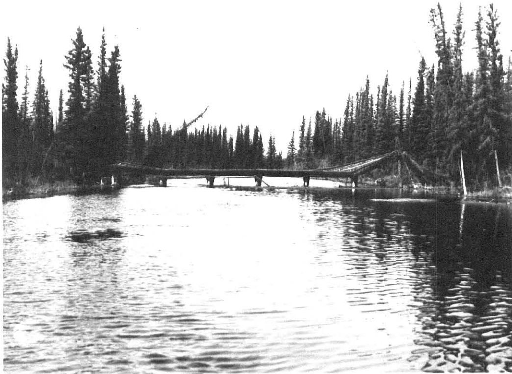
Fig. 9. Frost heaved piling of bridge spanning outlet of Clearwater Lake, southeast of Big Delta. Piles are wooden. Photo courtesy Department of the Interior.
