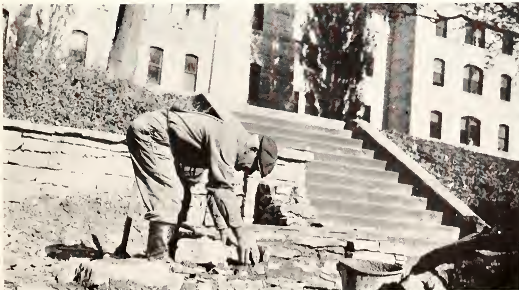
Working on Landscaping Project
