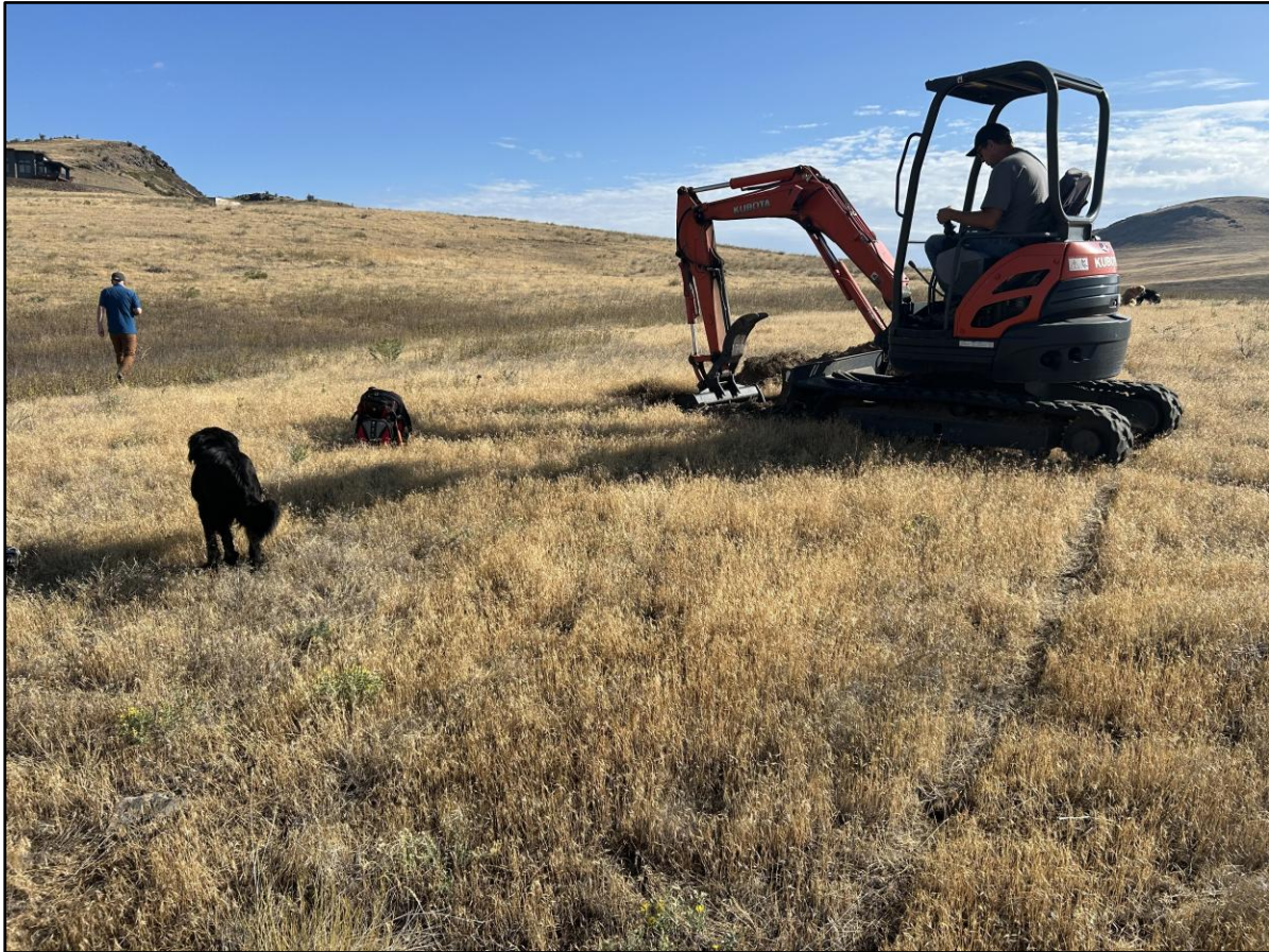
Figure 2.3: Image of a trench being excavated located at WCP. Two trenches were excavated at this location. One trench being shown here (Trench #2) and one atop the crest of the ripple in the background (Trench #1). While no image of the excavator is shown, a trench was dug excavated at BGR using a similar Earth mover from a different landowner
