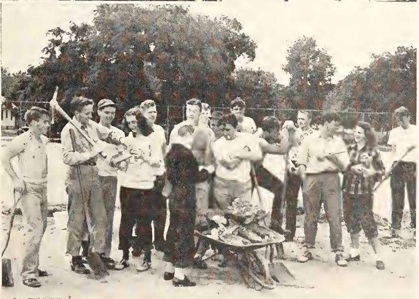
Men pitch in and work to clear the fences away for the new paved tennis courts on Hobo Day. The girls did their part by providing food and drink and a short break for the laborers.
