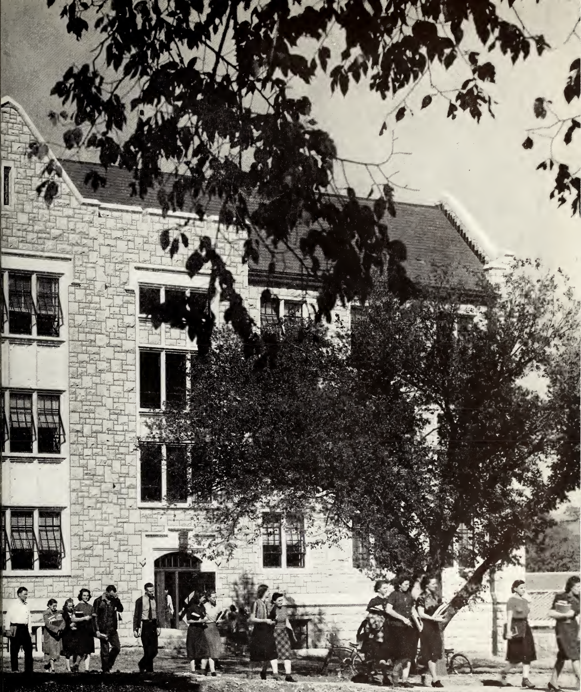
Willard's walls of native stone
