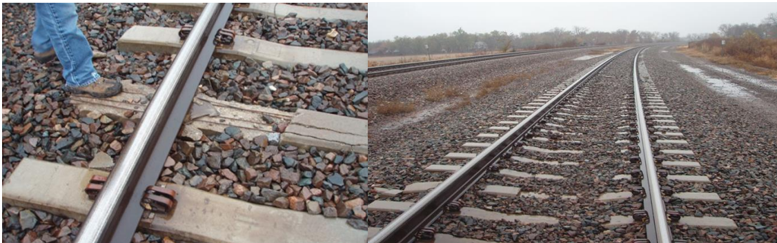
Figure 1-1: Failed Prestressed Concrete Ties
