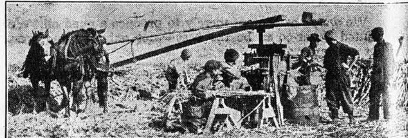
The Little Country Sorghum Mill Operated by Horse-Power Produces a Better Grade of Sirup Than the Large Mills for Several Reasons.
