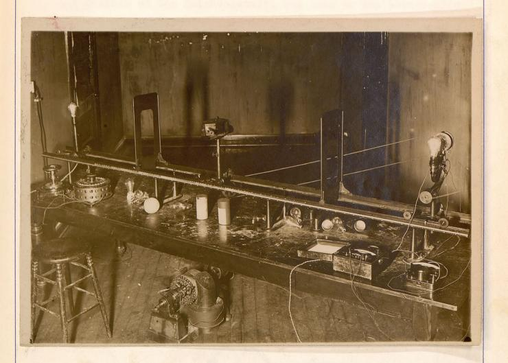
The scale extends the entire length of the photometer and is graduated both in centimeters and in candle power. The scale graduated in candle power is to be used only when the standard lamp is of 16 candle power.
