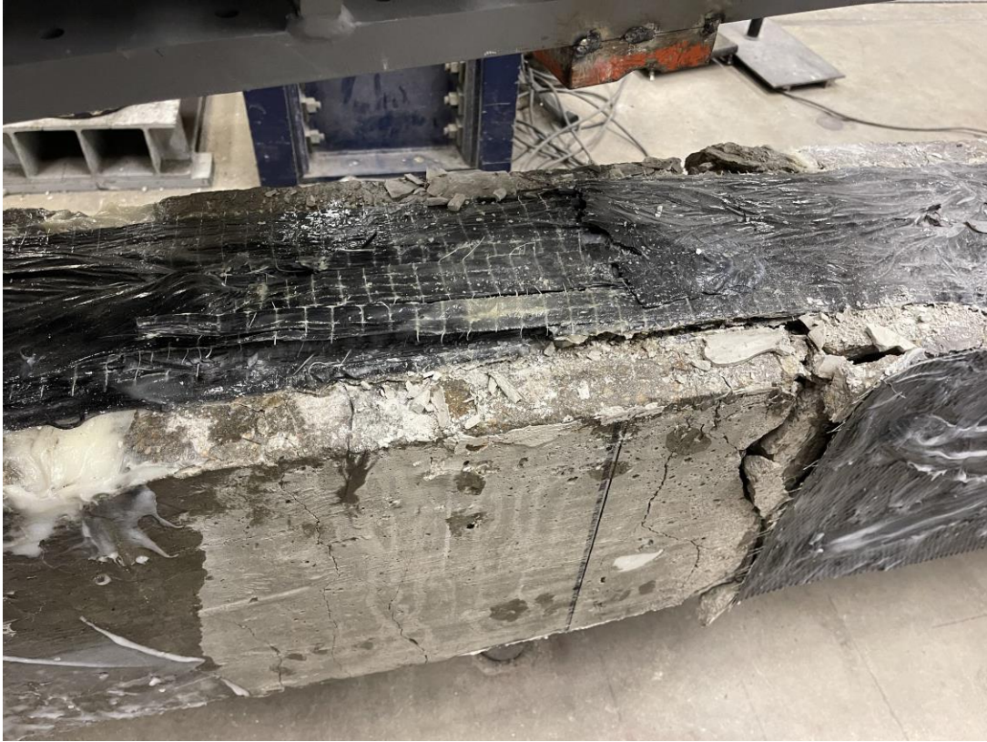
Figure 5.30. Failure mode of beam No.16.
