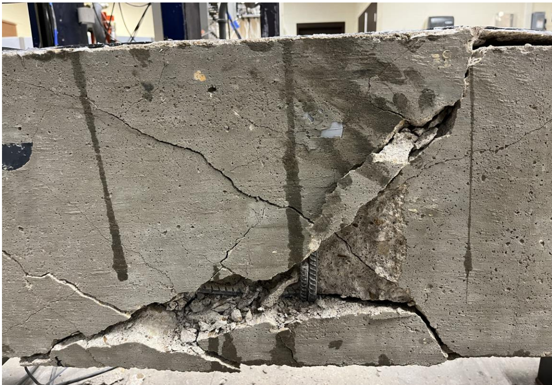
Figure 5.17. Failure Mode of beam No.6 due to shear cracks.
