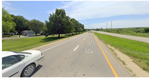
Figure 2.13: Looking South on Tuttle Creek Boulevard, Google Map's suggested walking route from Colonial Gardens to Walmart - pedestrians are forced to walk in the median or the ditch. Image screen captured from Google Maps.
