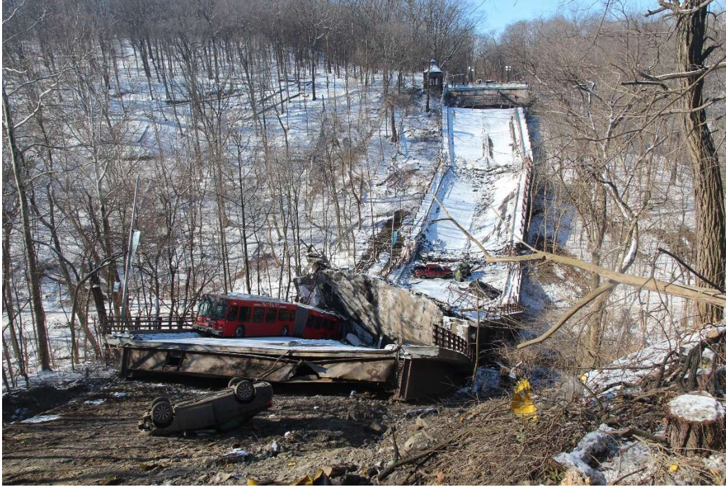
Figure 1.1: Fern Hollow Bridge collapse in Pittsburgh, Pennsylvania (2022) (NTSB, 2024)
