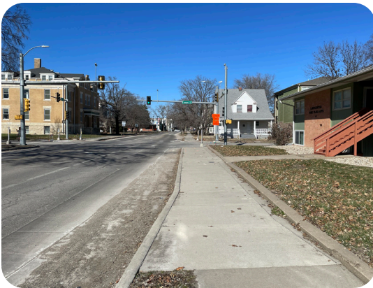
Figure 5.30 Newly-implemented bike lane and sidewalk on northwest corner (Skabelund 2024).
