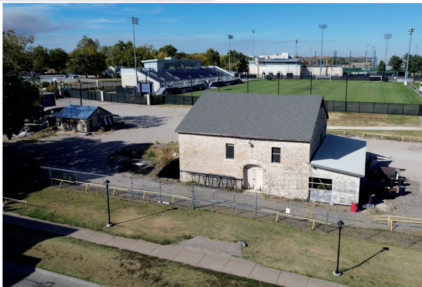
Figure 2.6: Aerial image of the Marlatt's barn and chicken coop, looking northwest. Photographed with drone by Andrew Littlefield
