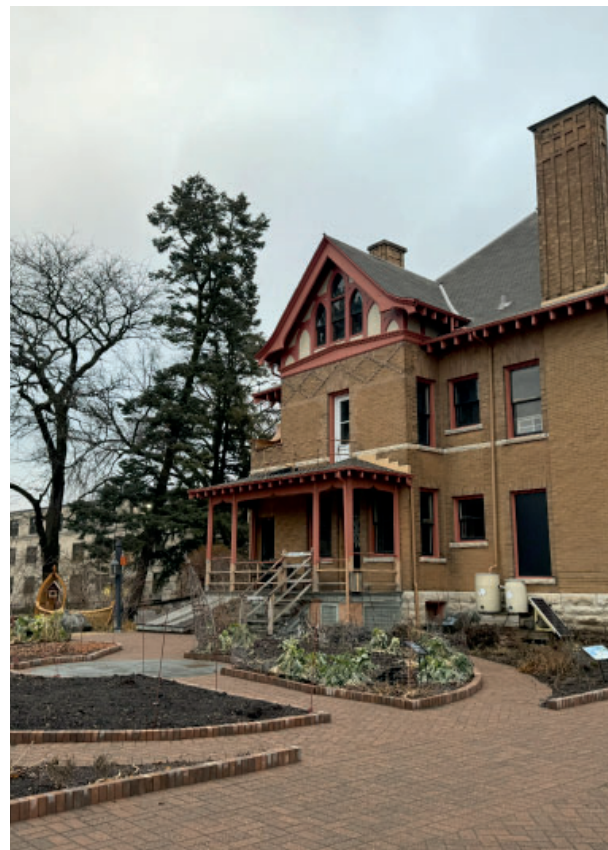
Figure 3.7: This entryway is lined with permeable pavers and garden plots and cisterns, showing the level of detail for water retention on the site. Photograph by Kate Lennon
