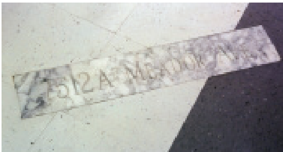
Figure 4.17 School Hallway (Rogers 2002)
