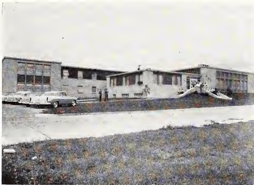
A $200,000 structure built in 1956 is home for 71 Alpha Kappa Lambda fraternity men at 1919 Hunting avenue.
