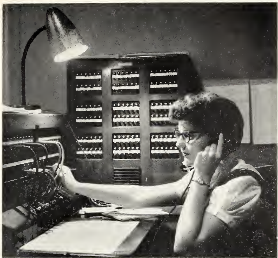
Working at the dorm switchboard provides a handy source of income for this Southeast hall resident.
