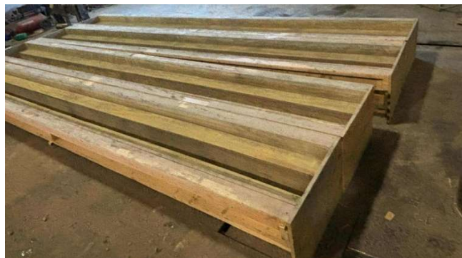
Figure 3.5: Wood formworks
