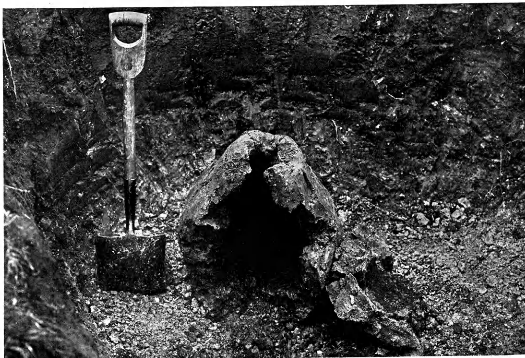
CAVITY PRODUCED BY DYNAMITING IMPERVIOUS SUBSOIL
