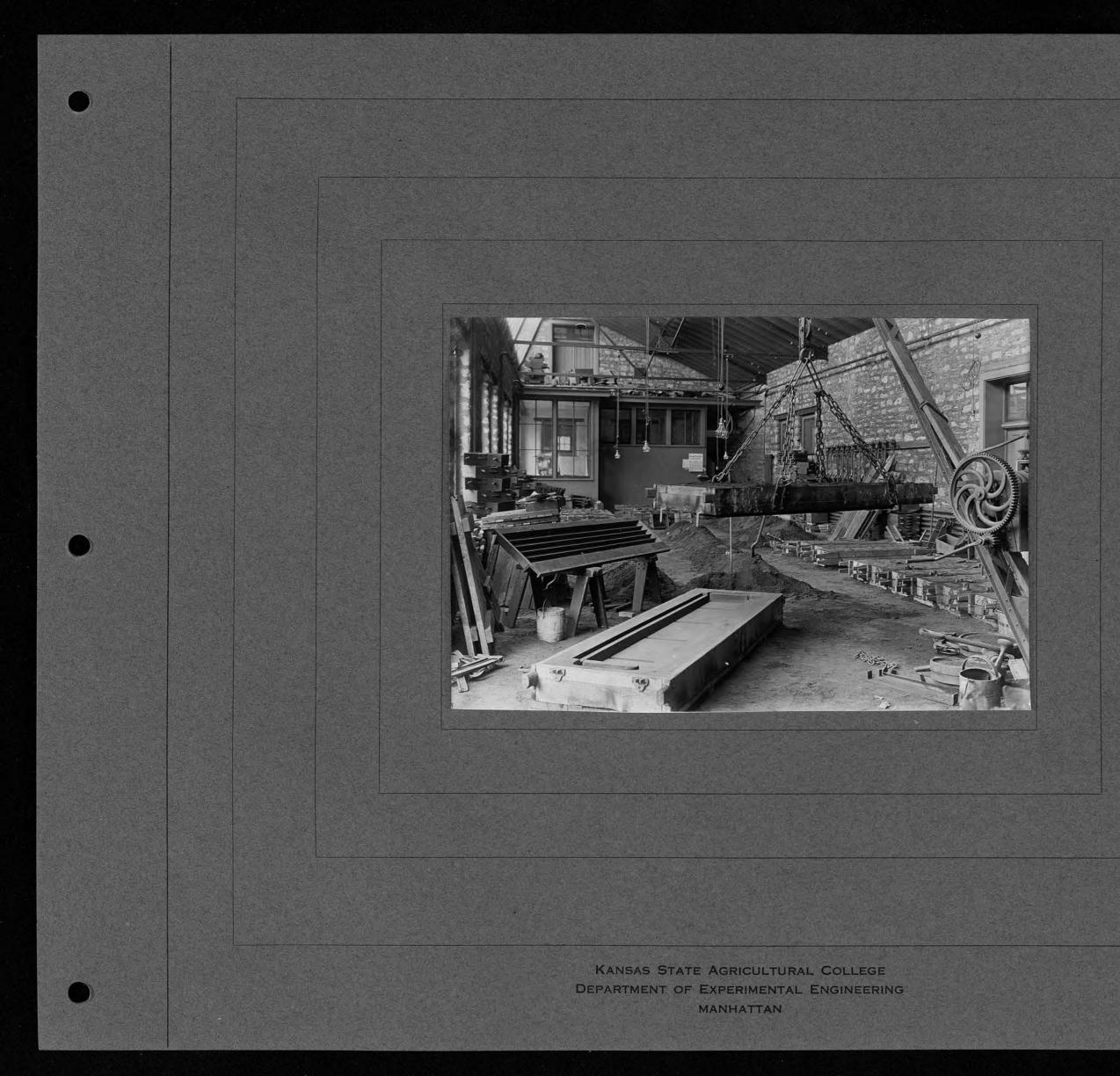
FILE No. SUBJECT: PATTERN & MOLD FOR JONES' STOKER DEAD PLATE (PATTERN MAREIN SHOPS) PLACE KSAC. FOUNDRY 5-40 DATE 1/12/11 12:00 1001 PLATE SEED 27.X BACKED LENGTH EXPOSURE \_\_\_\_\_M. \_\_\_\_S. STOP F. U. S.24 LENS DOUBLE FAL FOCUS CONDITIONS: DAYLIGHT FLASH LIGHT INTENSE SUN BRIGHT SUN HAZY SUN CLOUDY, BRIGHT CLOUDY, DULL NEGATIVE NO. U-55. LOCATION K.S.A.C. FILE PHOTOGRAPHER /
