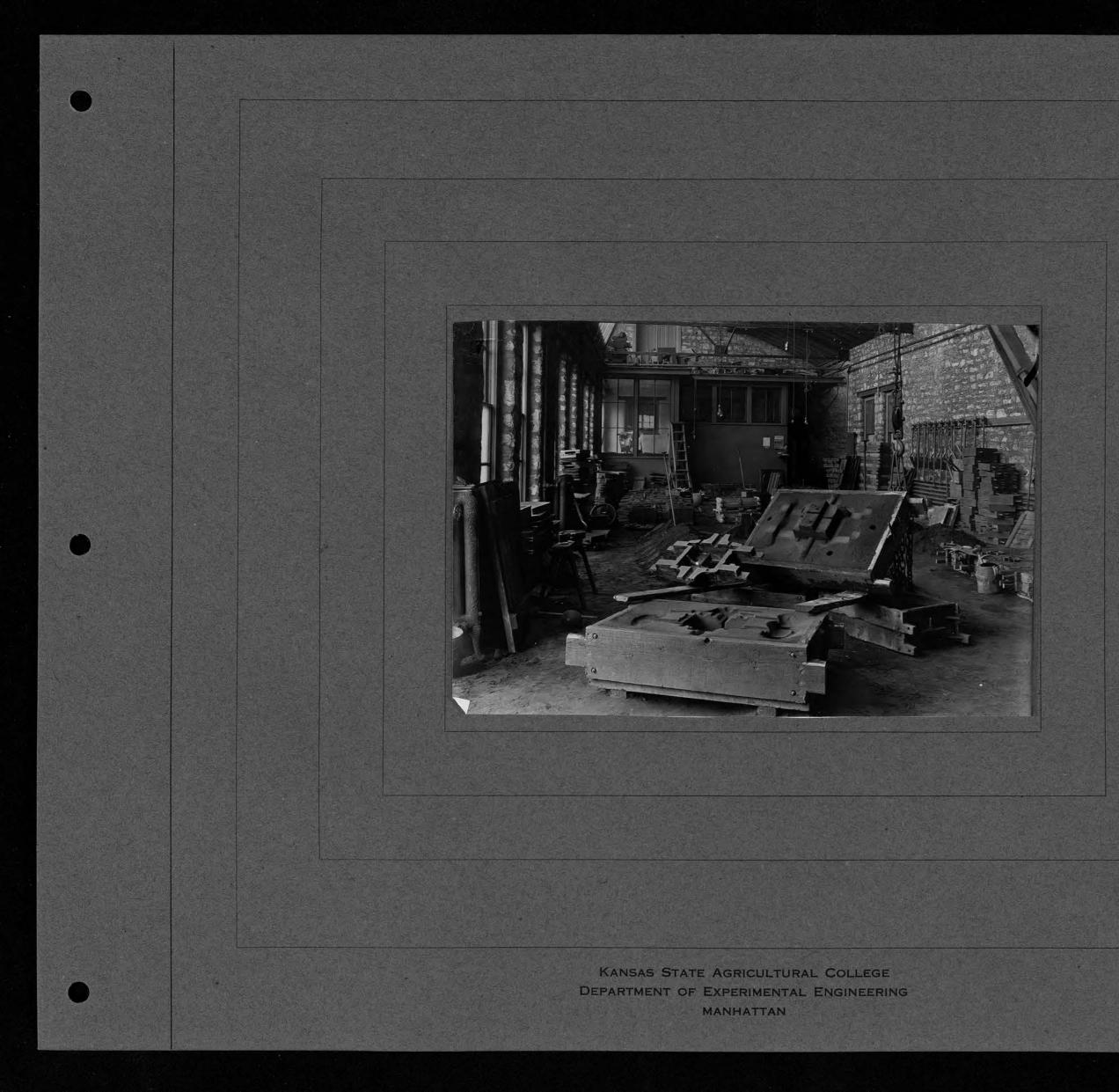
FILE No. SUBJECT: PATTERN & MOLD OF AUTO-MOBILE CRANK CASE. (STUDENT WORK) PLACE K. S. A.G. FOUNDRY 5-40 DATE 12/31/10 A.M. PLATE SEER 27x BAY FILTER LENGTH EXPOSURE 19 M. 30 S. STOP | F. 21..... LENS DOUBLE #4 FOCUS CONDITIONS: DAYLIGHT A FLASH LIGHT INTENSE SUN FLASH CART-RIDGE . BRIGHT SUN HAZY SUN CLOUDY, BRIGHT CLOUDY, DULL NEGATIVE NO. U-51 LOCATION K. S.A.C. FILE ..... PHOTOGRAPHER
