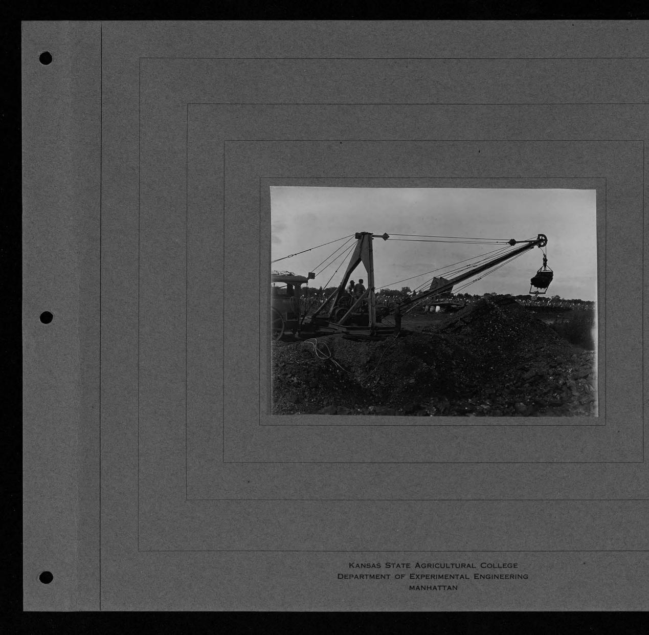
FILE No. SUBJECT: COAL PLT FIRE, REMOV ING COAL WITH AVERY" STEAM SHOVEL PLACE W. OF BOILER HOUSE DATE 123/11 10:45 A.M. PLATE SEED 27 X BACKED CONDITIONS: EXTERIOR INTERIOR DAYLIGHT FLASH LIGHT INTENSE SUN BRIGHT SUN HAZY SUN CLOUDY, BRIGHT CLOUDY, DULL NEGATIVE NO. U-38 LOCATION M.S.A.C. FILE -PHOTOGRAPHER
