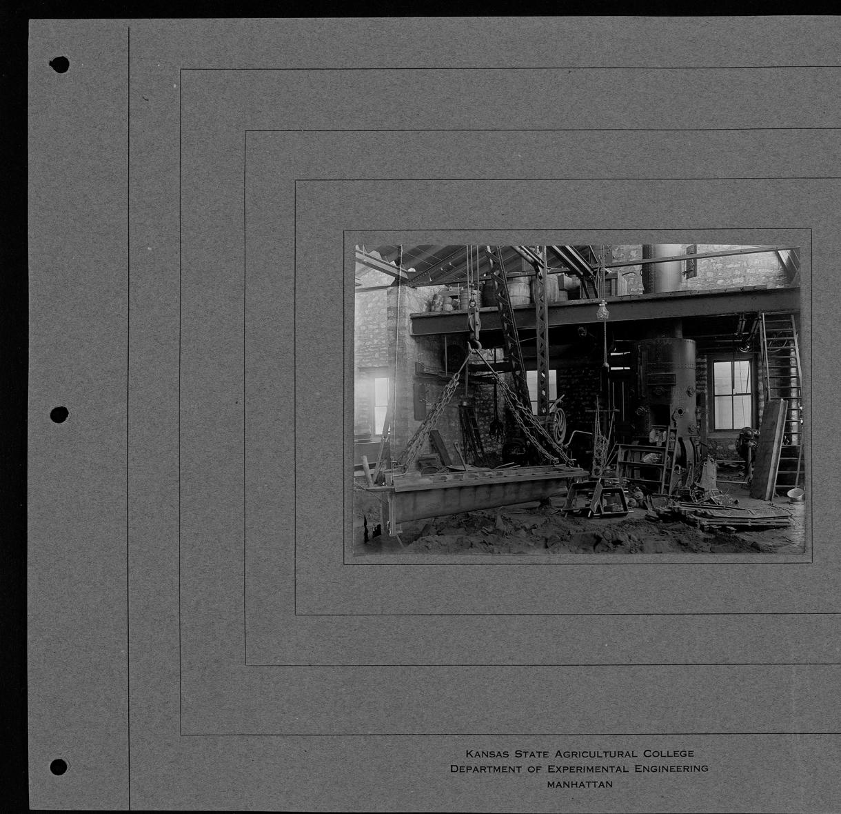
FILE NO. SUBJECT: CASTINGS BROKEN OUT OF MOLDS READY FOR CLEANING. PLACE M.S.A.C. FOUNDRY 5-40 (7:00 A.M. DATE \_\_\_\_\_\_\_ ..... P.M. AY FILTER PLATE SEED 27X LENS CONDITIONS: DAYLIGHT \_\_\_\_ FLASH LIGHT INTENSE SUN BRIGHT SUN HAZY SUN V CLOUDY, BRIGHT CLOUDY, DULL NEGATIVE NO. U-57 LOCATION M.S.A.C. FILE ..... PHOTOGRAPHER
