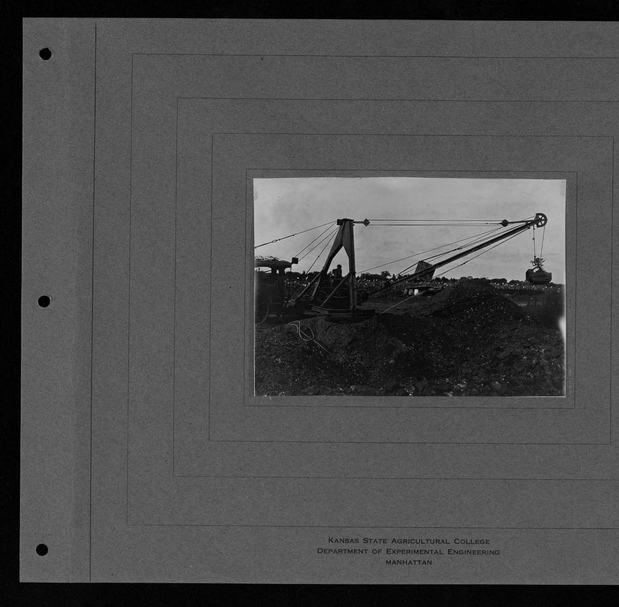
FILE No. SUBJECT: COAL PLI FIRE REMOV ING COAL WITH AVERY STEAM SHOVEL PLACE M. OF BOILER HOUSE PLATE SEED 27x RAY FILTER LENS DOUBLE FOCUS CONDITIONS: EXTERIOR INTERIOR DAYLIGHT FLASH LIGHT INTENSE SUN BRIGHT SUN HAZY SUN CLOUDY, BRIGHT CLOUDY, DULL NEGATIVE NO. U-36 LOCATION H. S. A. C. FILE ..... PHOTOGRAPHER
