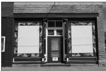
Glasco Storefront Restoration.
