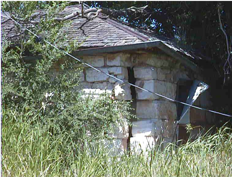
Figure A2.12. Structure is composed of KS-26. This structure was located on the property of an abandoned pit-quarry where KS-26 was mined. Unable to locate the abandoned pit-mine due to overgrowth of flora. Current work suggests KS-26 is genetically similar to Lava Creek B Tuff of the Yellowstone Caldera. Picture was taken by Van Fleet, 1999.
