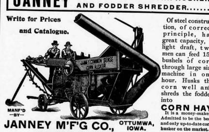
Of steel construction, of correct principle, has great capacity, is light draft, two men can feed 150 bushels of corn through large size machine in one hour. Husks the corn well and shreds the fodder into
