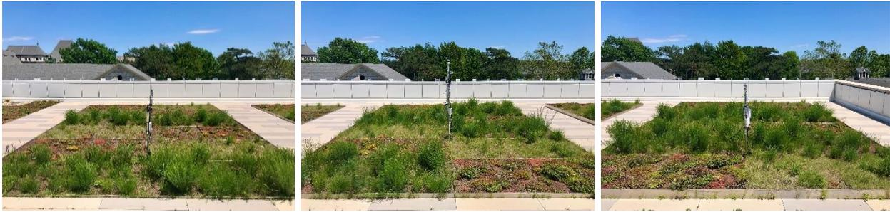
**Figure 1.3.** Photos of the three APD-EGR beds (4-, 6-, and 8-inch deep, shown from left to right, respectively) APD-EGR.
