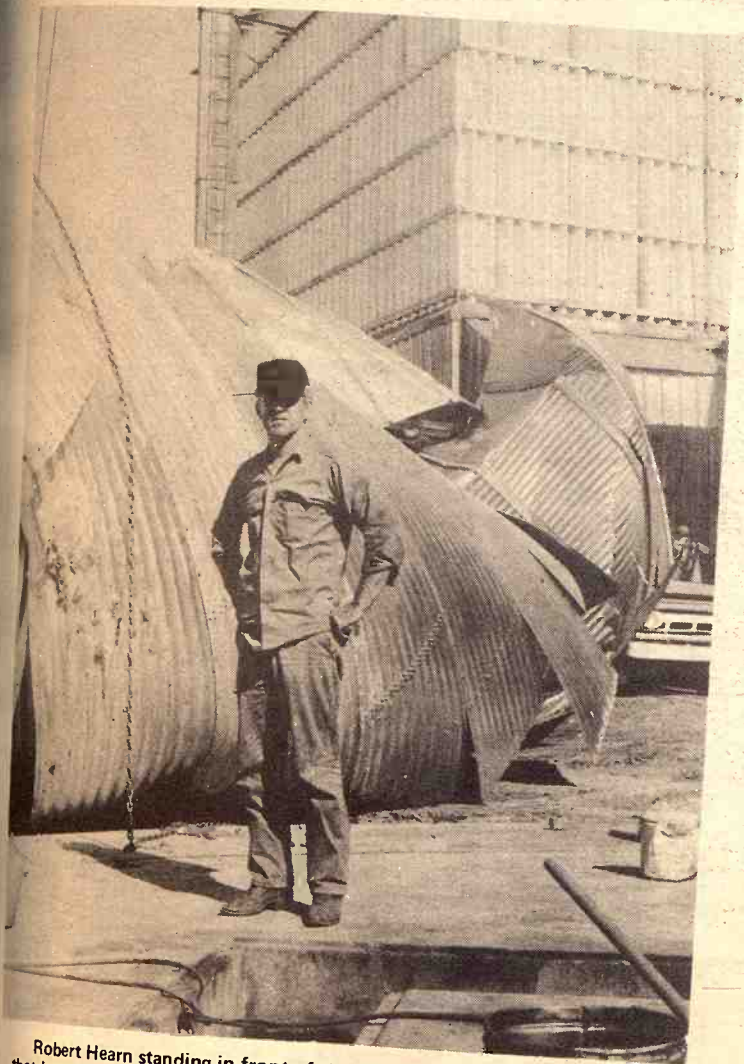
Robert Hearn standing in front of the remains of a 72-foot grain bin that Lamoreaux Construction Co. was building at the Waterville Co-op. They lacked just a few feet of having it finished when it was blown down. It was the only building at the co-op that fell to the high winds.
