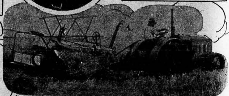
C. W. Sheldon, of Henderson County, Illinois, Encountered Soft Soil During Wheat Harvest, so He Put 36-Inch Extension Lugs on the Tractor Drive Wheels and Placed a Plank Under the Bull Wheel of the Binder and Went Ahead
