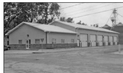
Axtell Emergency Services Building
